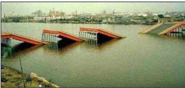
**Fig.5:-Failure of the Showa Bridge after the 1964 Niigata Earthquake.**
